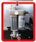
Step 3) Remove Top and bottom bolts from trash door actuator.
